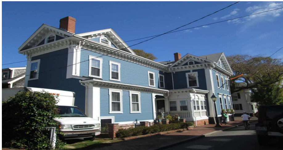
REAR OF SUBJECT
